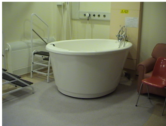
Photograph 23 Non slip flooring around a birthing pool
